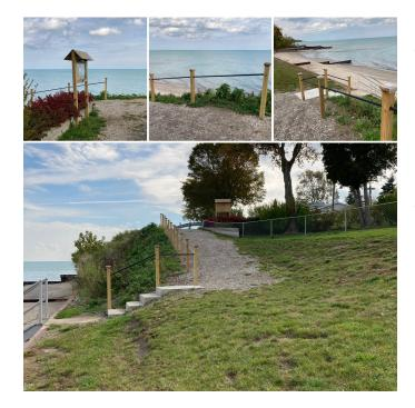
The access at Huron Bay beach was graded and shaped, fixing an erosion problem, and finishing it off with grass seeding and a handrail and stairs.
